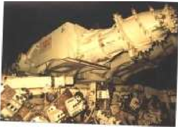
side view of the new booms added on top of the base Marietta miner!
